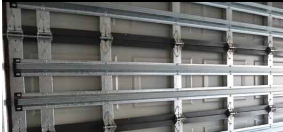
Double end stiles and additional centre stiles for maximum strength.
