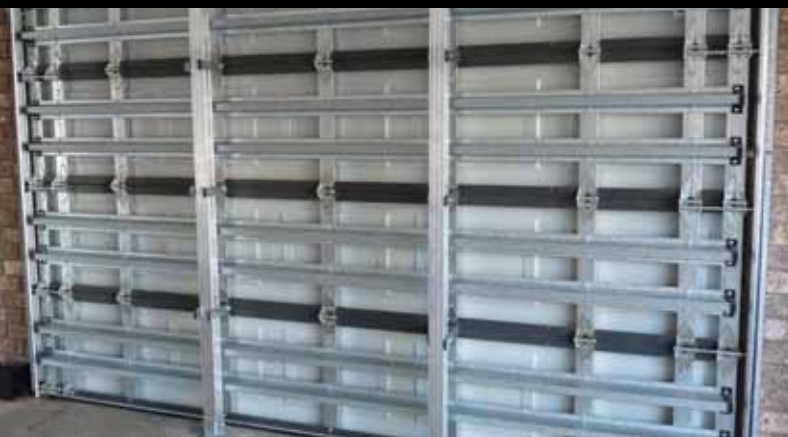
Internal view with bracing system secured.
