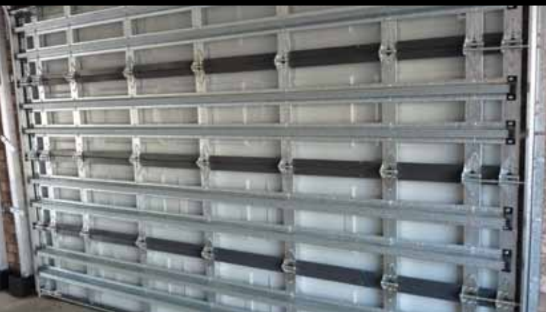
Internal view without braces secured.
